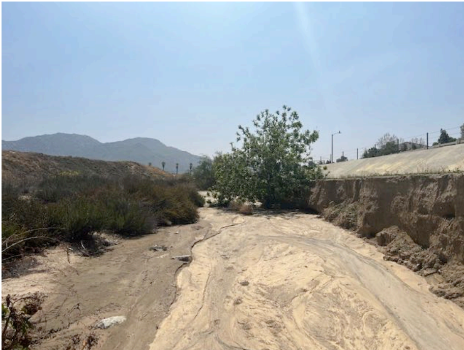
Photograph 6: South-facing view of channel in Reach 2 from Photo Point 6.
