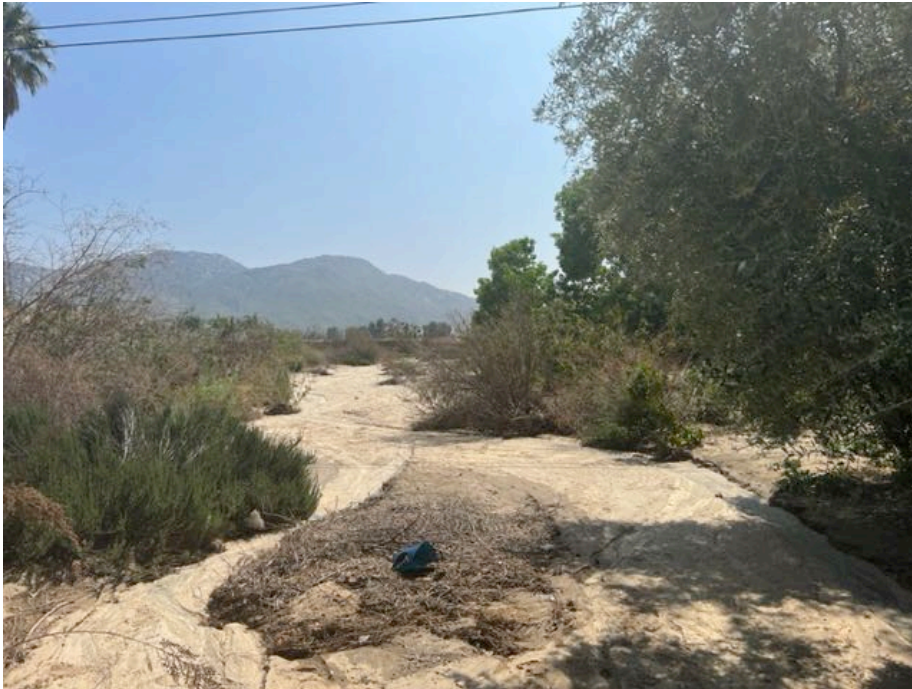
Photograph 15: South-facing view of channel through Reach 5 from Photo Point 15.
