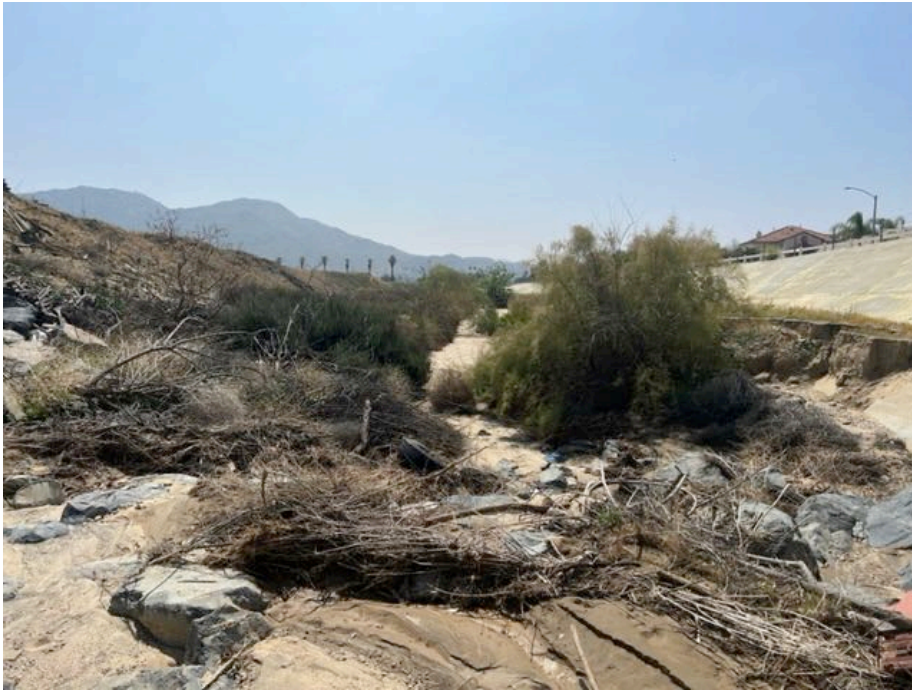
Photograph 3: South-facing view into Reach 2 from Photo Point 3. Riprap in the photo foreground is at the southern boundary of Reach 1.
