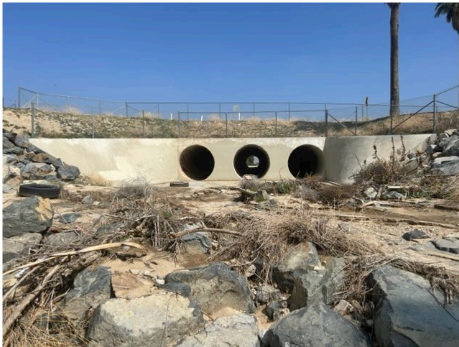
Photograph 2: North-facing view from Photo Point 2 at the southern boundary of Reach 1.
