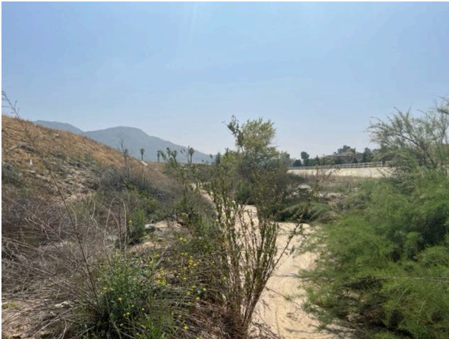
Photograph 8: South-facing view of channel in Reach 3 from Photo Point 8.
