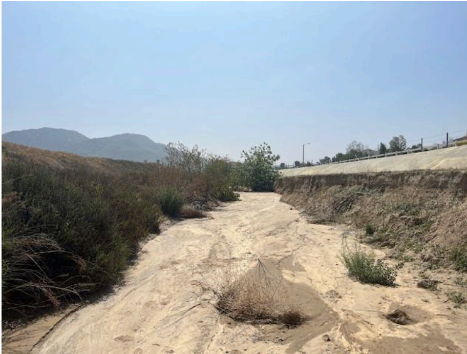
Photograph 5: South-facing view of channel in Reach 2 from Photo Point 5.
