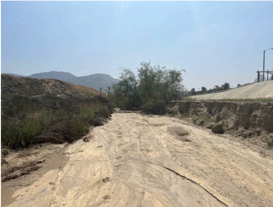
Photograph 7: South-facing view of channel in Reach 3 from Photo Point 7.
