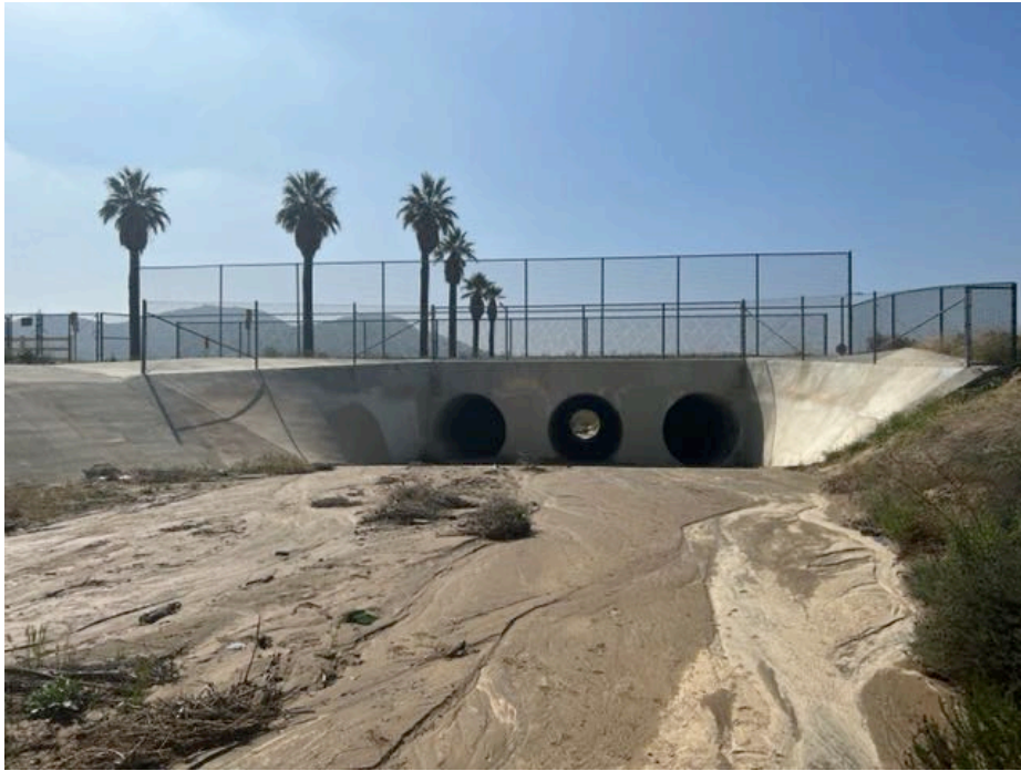
Photograph 1: South-facing view of Reach 1, from Photo Point 1, where three concrete-encased culverts pass under Cottonwood Avenue.
