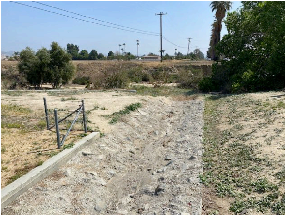
Photograph 30: East-facing view of concrete swale that runs east-west at the south end of the intersection of Bay Street and Quincy Street, ultimately emptying into Reach 5 of the channel.
